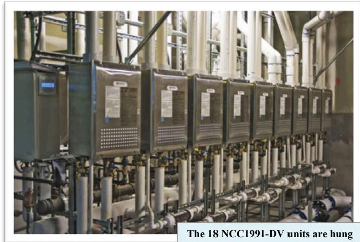
The 18 NCC1991-DV units are hung and piped together in a 16-ft. x 7-ft., custom-fabricated, Unistrut rack system located in a 1,000-square-foot, “penthouse” mechanical room on the roof of the AVA 55 Ninth building. The high-efficiency, condensing models all have an Energy Factor of 0.95
