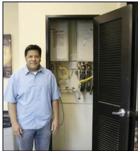
Greg Paulino with two of the condensing type tankless water heaters that were installed in the laundry rooms at Vintage Crossings. Paulino says he saved “between \$200 and \$300 on material costs for each of the two installs” by using PVC venting rather than stainless steel.
